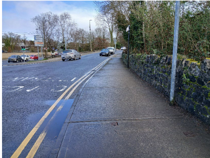
Plate 5 Looking north along Southern Station Road.
