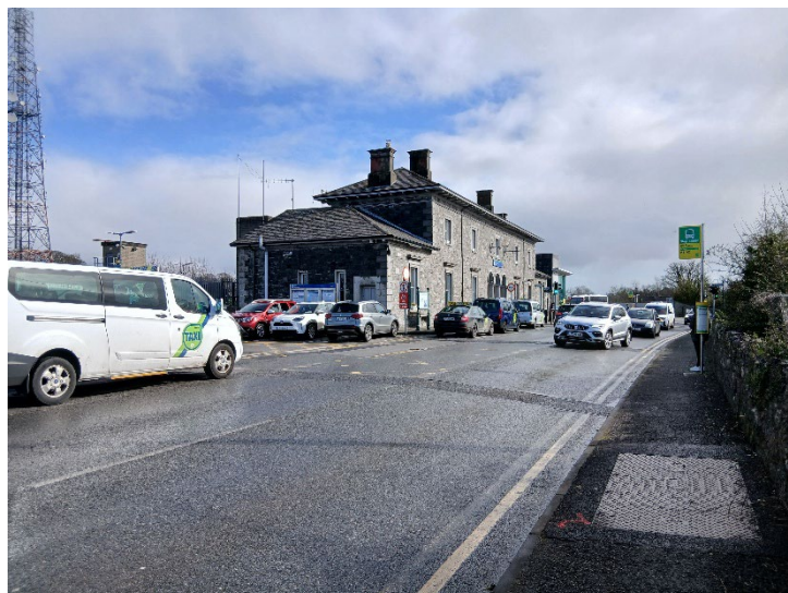
Plate 6 Looking east along Southern Station Road showing Railway Station (RPS 145).
